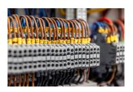
Control Cables: Used to connect control devices such as sensors, switches, and actuators to controllers. Essential for the efficient operation of automated systems.
